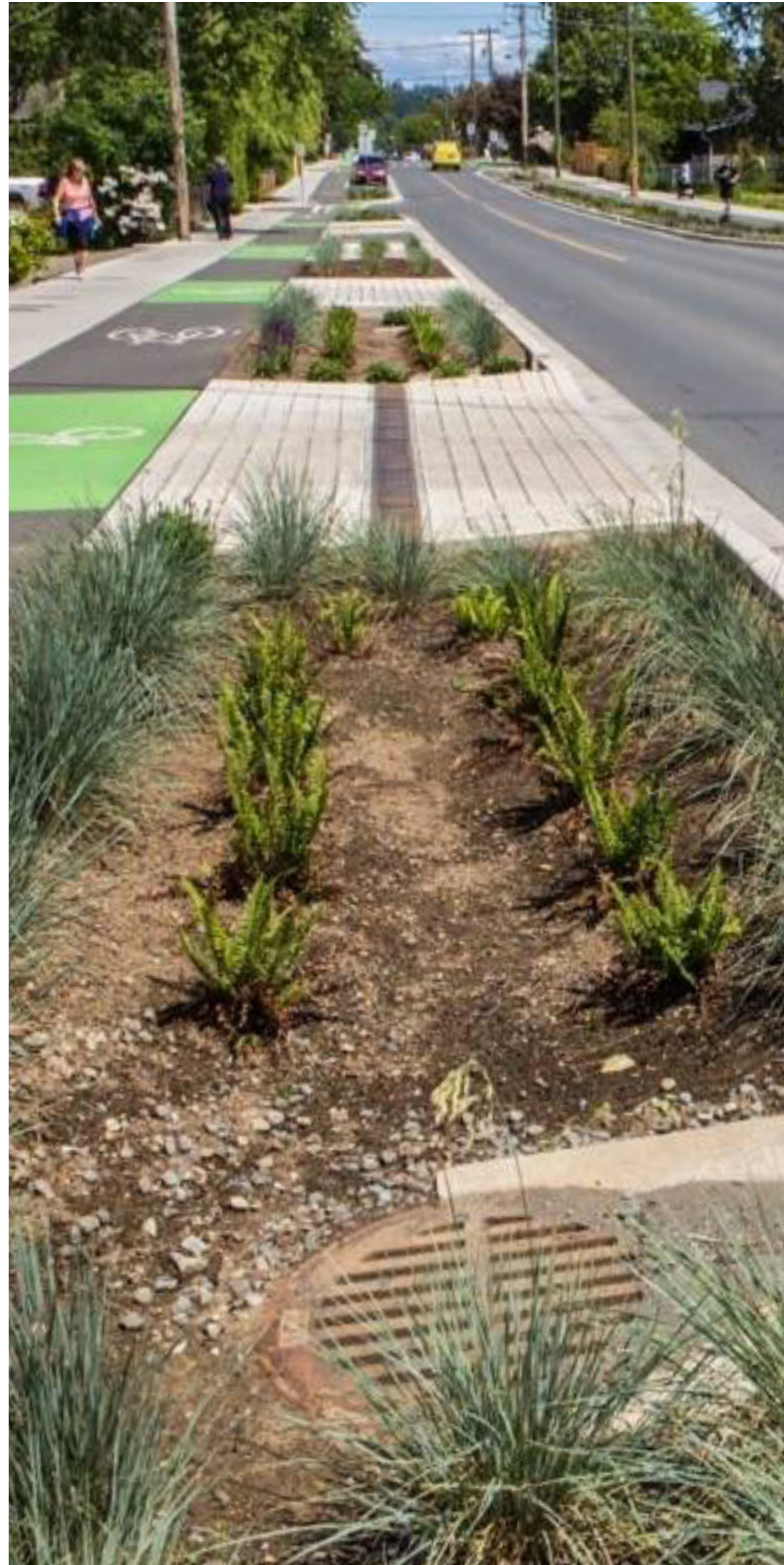
Image: 5th Street Complete Street Integrated Rainwater Management.
